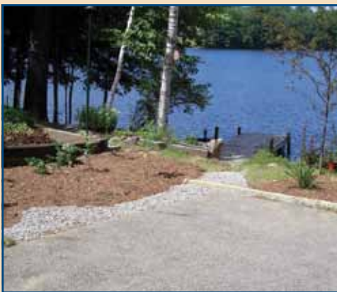
Before (top) the LCC crew visited this property at Clough Pond, runoff flowed directly off of the driveway and into the pond. After the crew visited (bottom), several BMPs had been installed to reduce the runoff.
